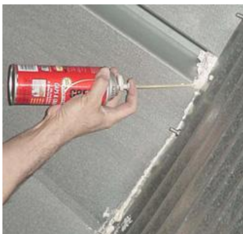
Sealing seams with silicone caulk (photo: factsheets.okstate.edu)
