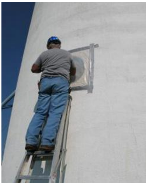
Sealing opening (photo: Oklahoma State University)
