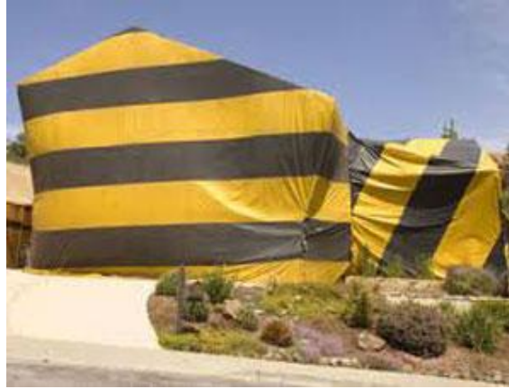
Structural fumigation (photo: sanjoaquinpestcontrol.com)
