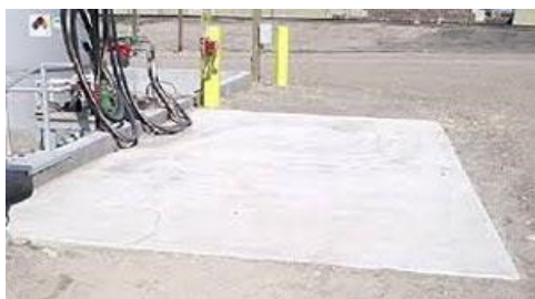
Impervious containment pad
