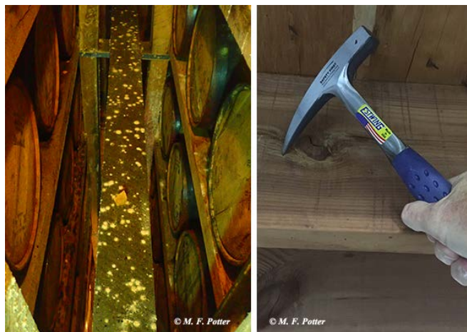
Substantial powder warrants further investigation. A pick hammer is useful when surveying for deterioration.
