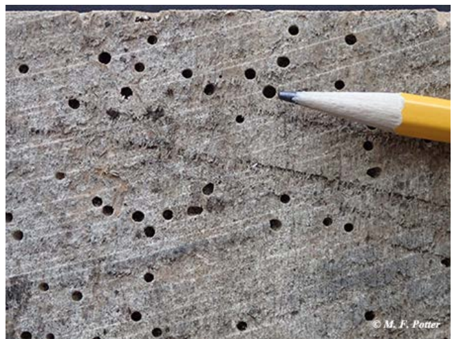
Old emergence holes suggesting infestation is no longer active
