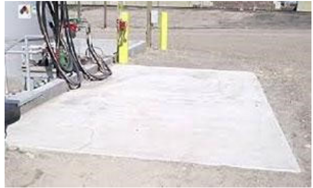
Impervious containment pad
